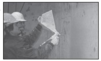
Apply second, stiffer consistency, coat of *Cem-Kote CW Plus* into the wet slurry by trowel. Keep wet edge. Do not build up a layer thicker than 6 mm (1/4 in). In new construction, *Cem-Kote CW Plus* is dry-sprinkle applied onto the surface of the freshly poured slabs (after the concrete starts to reach initial set) and is power trowel finished.
